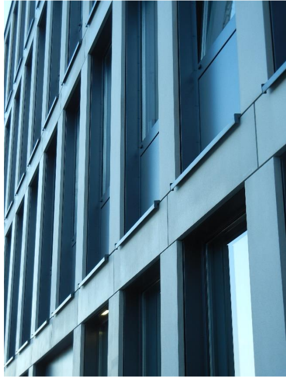
Façade made by Benno Drössler GmbH & Bauuntern. KG
