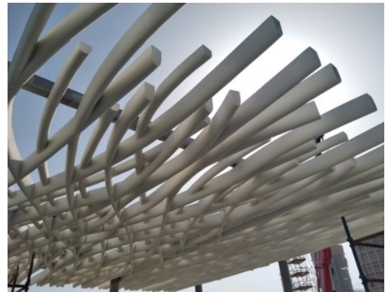
Shading roof for Lusail Plaza Qatar (© DCS/Ayman Badr)
