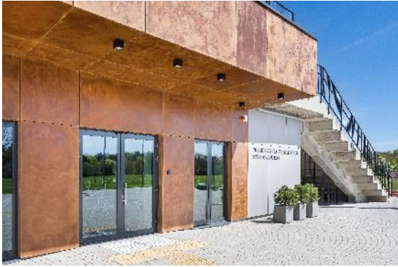
Two types of façade panels made by Hibeton, implemented at University Sports Center, Kaunas, Lithuania (© Hibeton)
