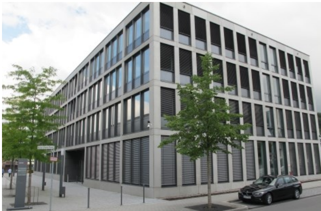
Cladding Façade in Germany by Drössler (© durcrete)
