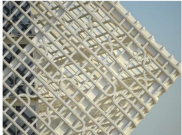
Structural elements and façade panels
