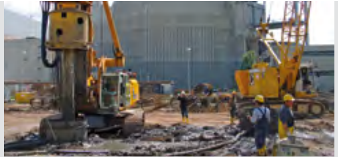
Pile drilling
