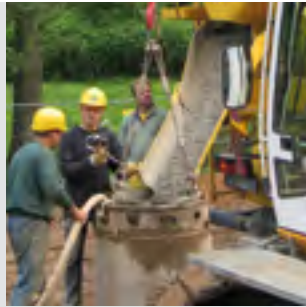
Filling the pile with concrete
