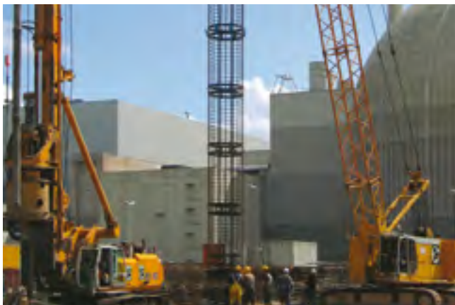
Concrete pile construction
